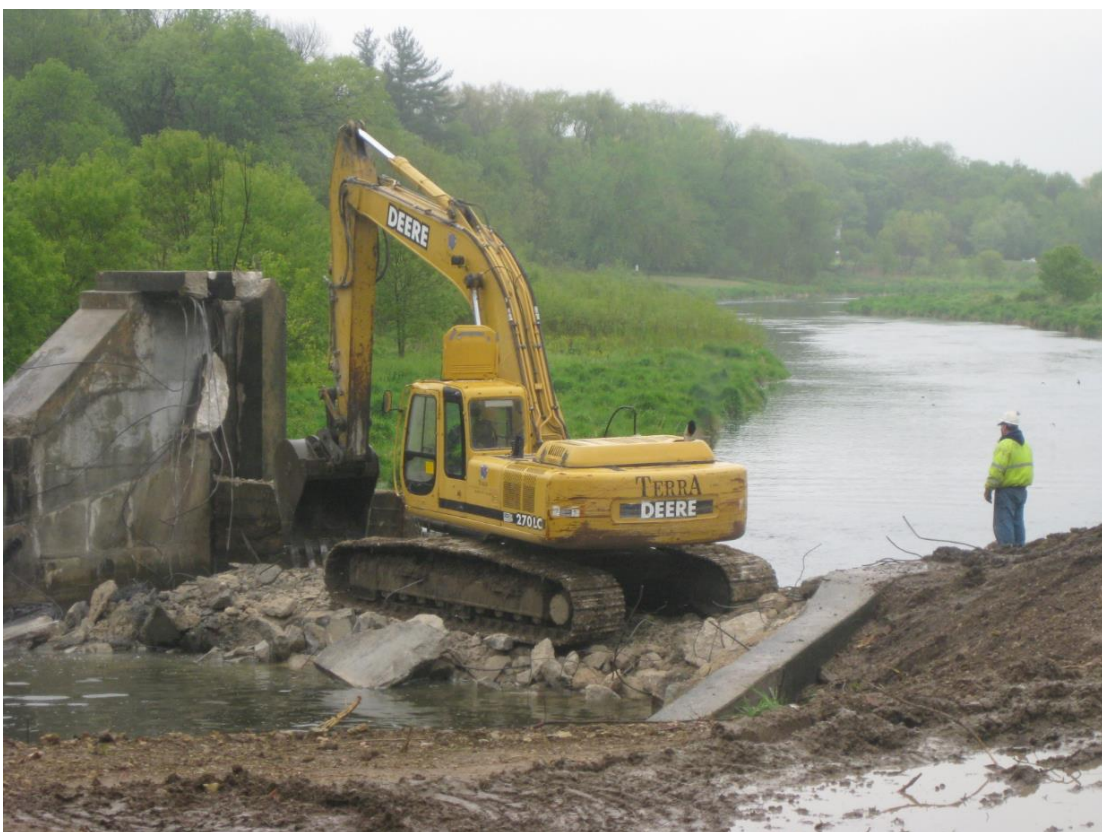
Stebbensville Dam Removal – May 2010
